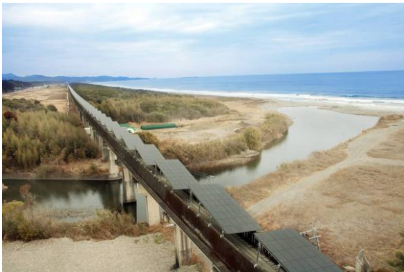
Photo 1: The second stage of Tsuno SolarWay built on a former maglev test track in southern Japan
