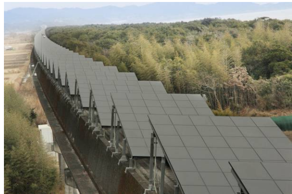
Photo 2: This time around construction methods and efficiency could be improved thanks to the trial results of the first stage.
